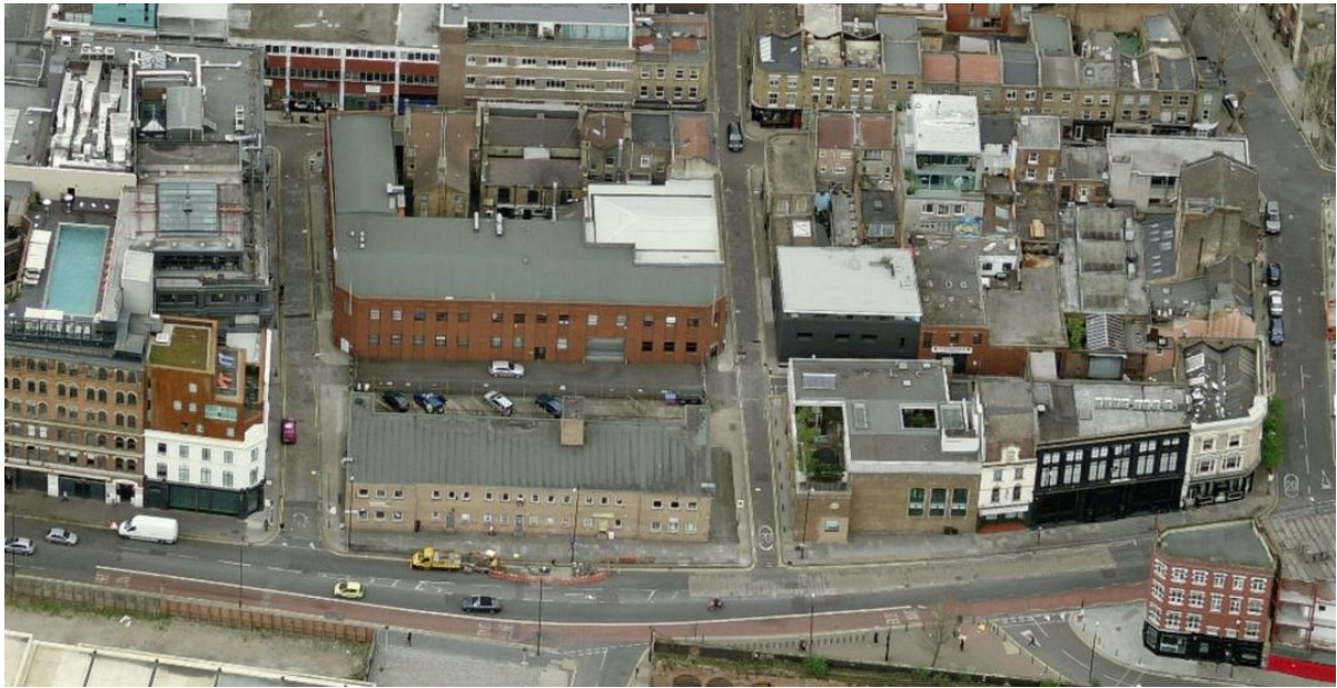
Figure 2: Birdseye view from the south (Source: Bing Maps)
