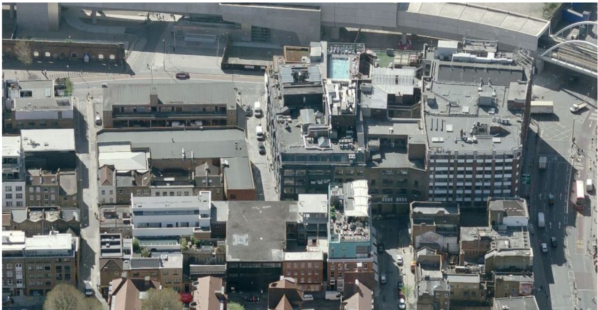
Figure 3: Birdseye view from the north (Source: Bing Maps)
